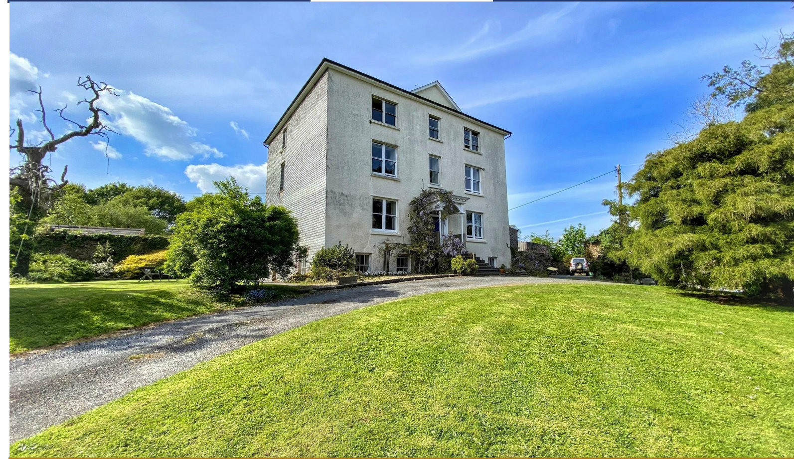
Begelly House Begelly, Kilgetty, Pembrokeshire, SA68 0XE
